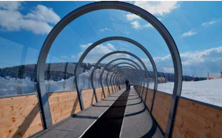
Ski tunnel in the Kopaonik ski area in Serbia, solid clear polycarbonate sheets, Polycasa® PC
