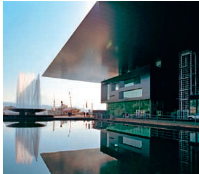
"Flying roof" of the Culture and Convention Centre Lucerne (KKL), constructed using Alucore composite panels from 3AComposites.
