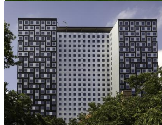
Union on 24th, Austin, Texas Architect: Perkins & Will Prefabricated elements
