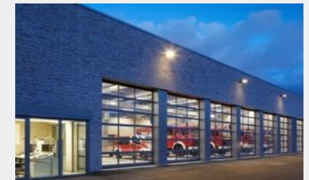
POLYCASA® SAN HC® Sectional garage doors made out of scratch resistant SAN sheets
