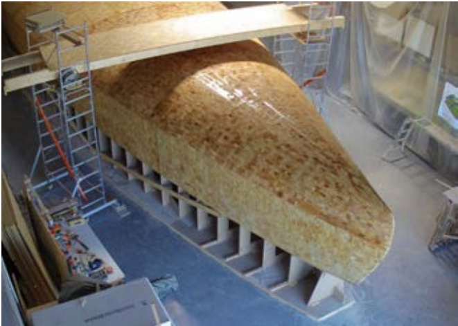
▼ Construction of INNOVATION YACHTS prototype Open60AAL
